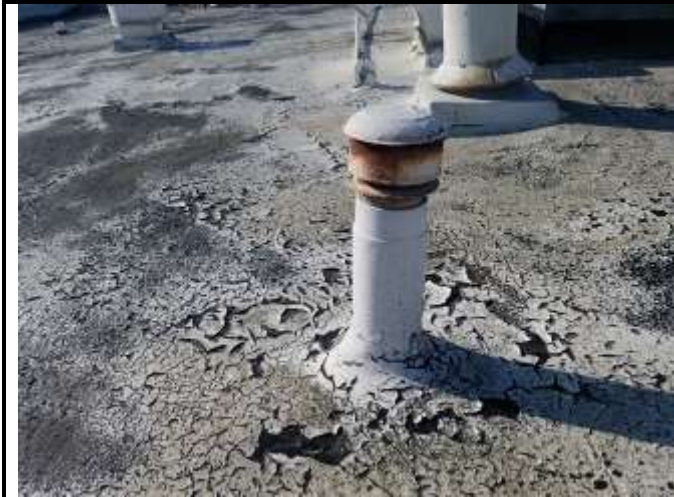
Photo 1: roof- transite vent pipes (ACM)
