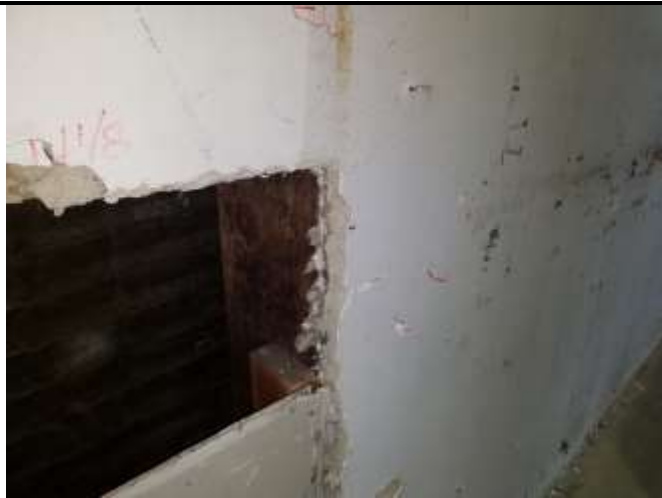
Photo 9: plaster system (non-ACM)
