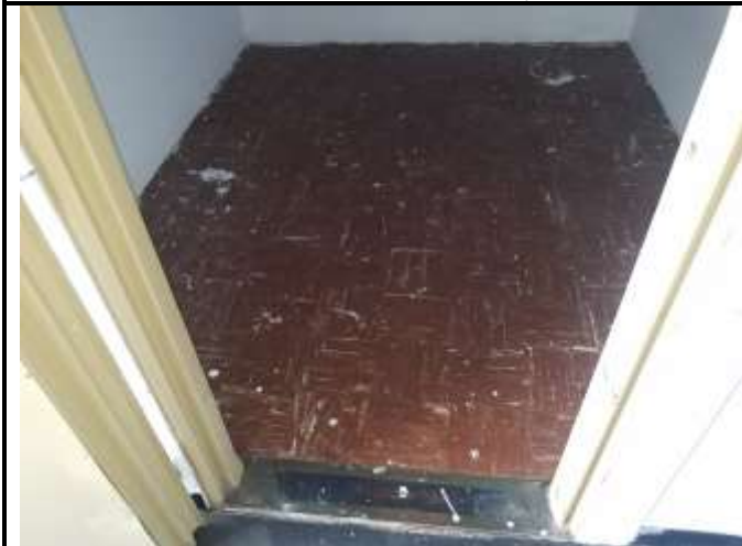
Photo 5: 2 nd floor vault and storage - brown 9”x9” VFT (ACM)
