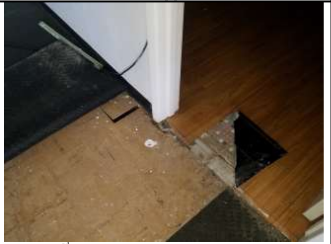
Photo 6: 2 nd floor main room and men’s bathroom – 9”x9” VFT (ACM) and ceramic floor tile (LBP)
