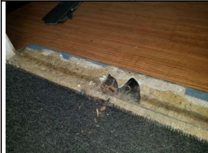
Photo 3: Women’s restroom floor – multilayer VFT (ACM)
