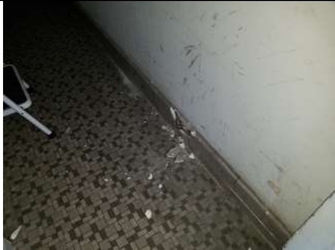
Photo 7: 1 st floor storage/electrical room wall and floor ceramic tile (LBP)
